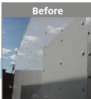
Before Previous process. Note the proliferation of rivet heads.
